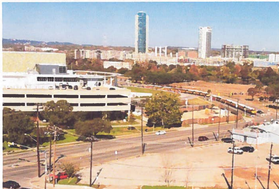
Figure 7: Existing Bus Staging on W. Riverside Drive
