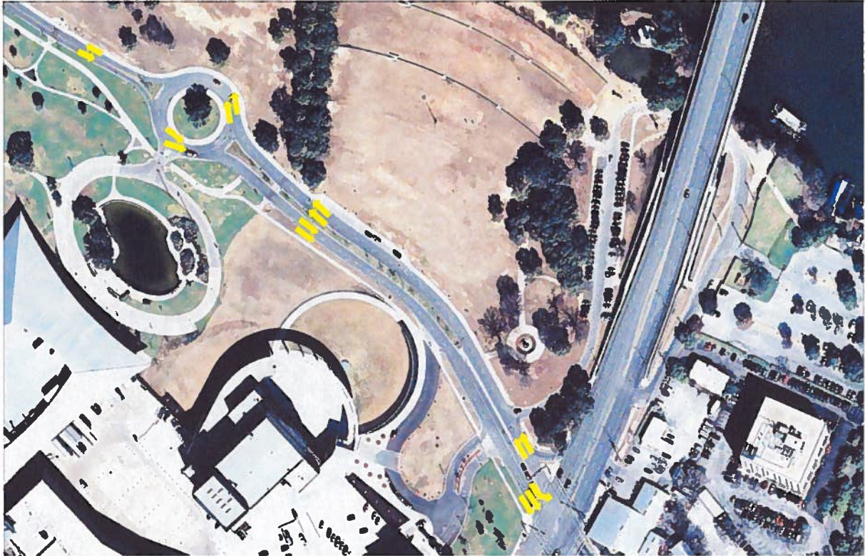
Figure 3: W. Riverside Drive between S. Lamar Boulevard and S. First Street
